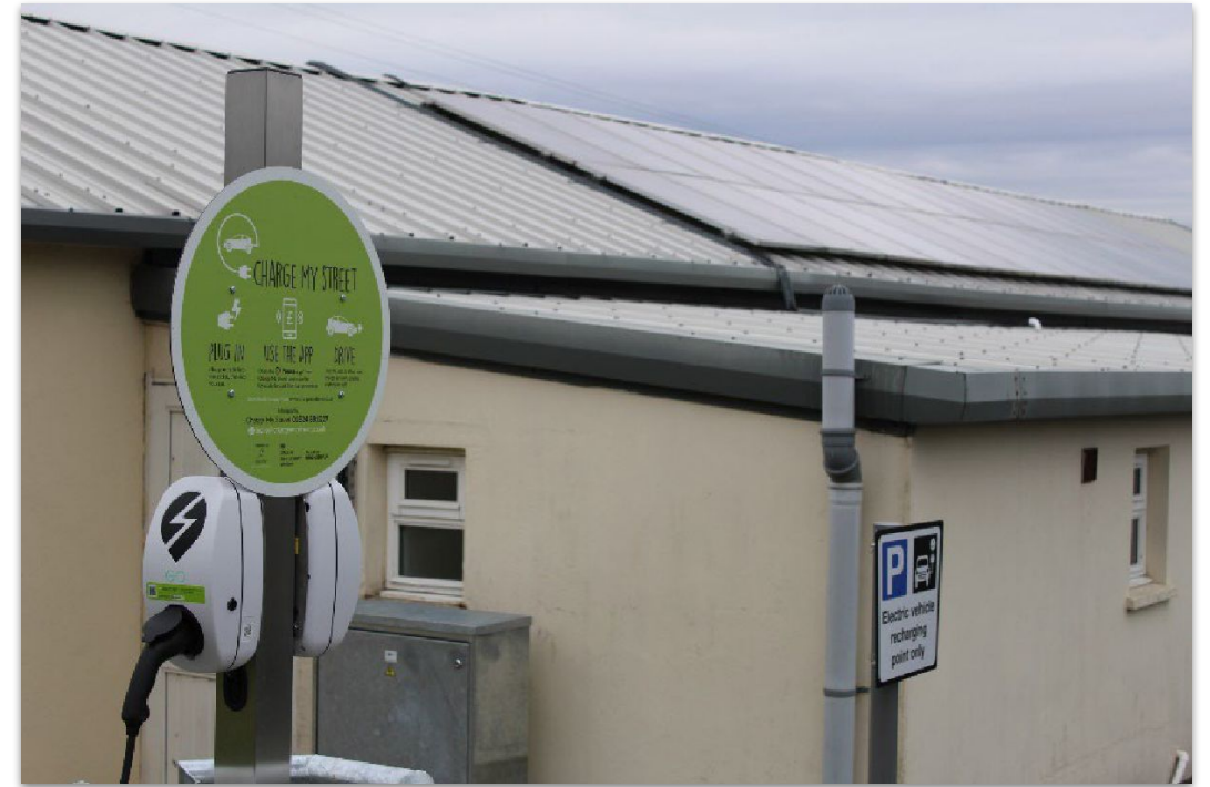
Solar Panels on Morland & Newb Village Hall, Penrith
